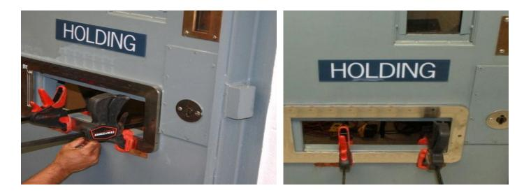
Next line up the PASS Door Frame to the cell door food port opening. Secure in place with clamps. KEEP BOTTOMS OF FRAME & PORT FLUSH AND SMOOTH.
