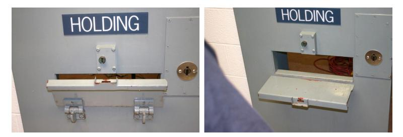
Above is a typical cell door metal plate drop-down food door that will be replaced with the PATENTED ANTI-SPLASH SYSTEM (PASS) Frame.
