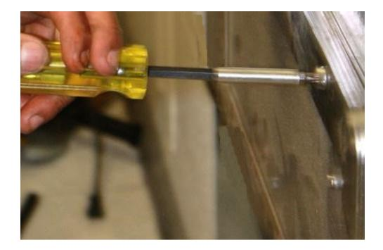
Secure the PASS Frame to the cell door using the Security Screws supplied with your PASS unit. It is HIGHLY recommended that a screw thread adhesive such as "Loctite" or similar adhesive product be used on the threads of the Security Screws to assure a secure bond.
