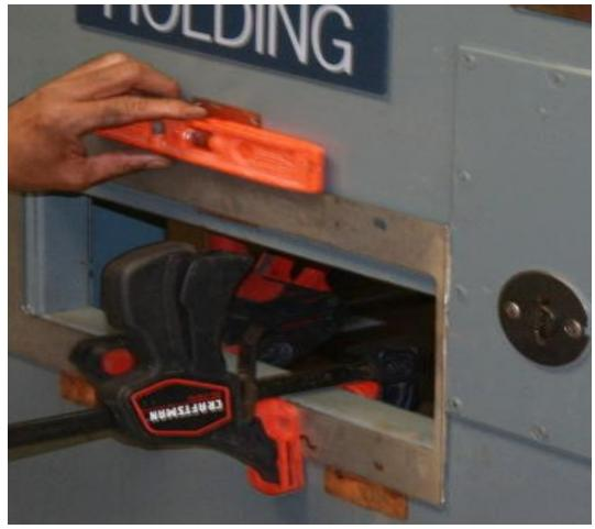
Make sure the bottom of the PASS Frame opening is level and in line with the <u>bottom</u> of the food port opening. Also make sure that both sides of the PASS Frame are evenly space with the sides of the food port opening.
