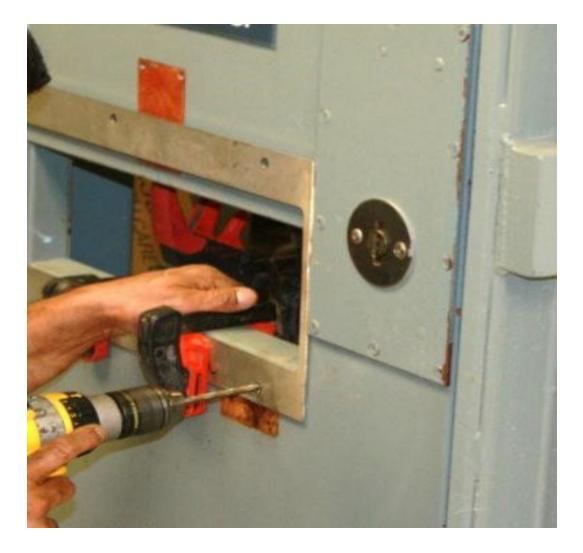
Drill and Tap the cell door according to the pilot screw holes in the PASS Frame. The recommended Tap size is  $\frac{5}{16}$  - 18 and Drill Bit F-.257. This Drill Bit and Tap combination should produce the proper size hole and thread for the security screws supplied with your PASS unit.
